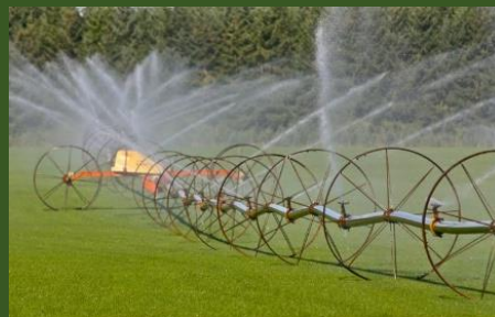
A wheel line sprinkler system.
